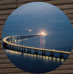
Hong Kong-Zhuhai-Macao Bridge
